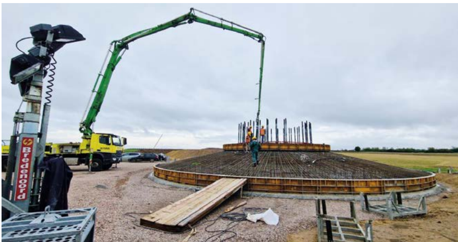
Windparkbau in Gau-Bickelheim.
